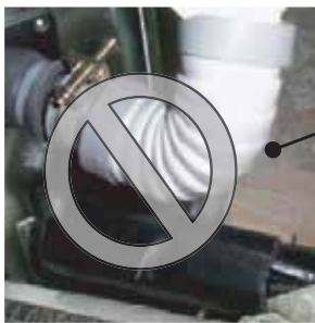
Figure 56: Condensate Drain Piping Should Not Include Sharp Bends.
