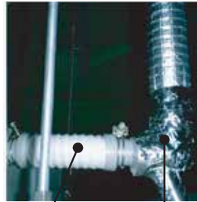
Figure 55: Properly Insulated Condensate Drain Piping.
