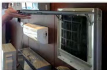
4. Lift front panel all the way. Be sure to hold with one hand at all times while removing filter.
